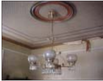
The parlor ceiling before restoration.
