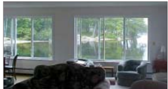
New windows offer better view, ventilation.
