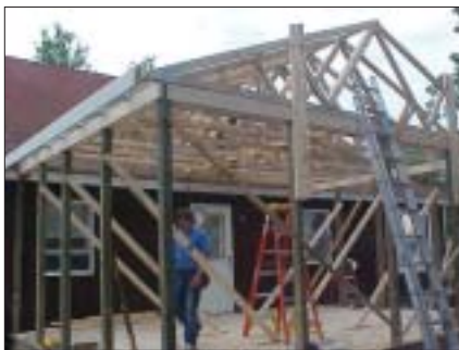
The porch under construction.
