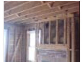
Mold removal work.
