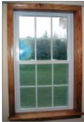
One of the new windows.
