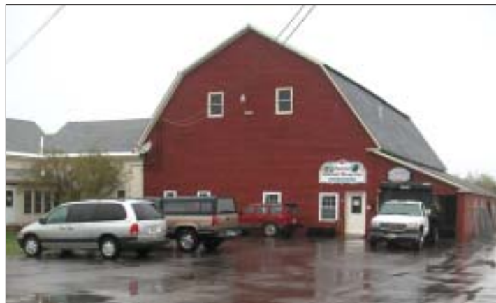
The Chester Animal Hospital was reconstructed in this 90-year-old barn.
