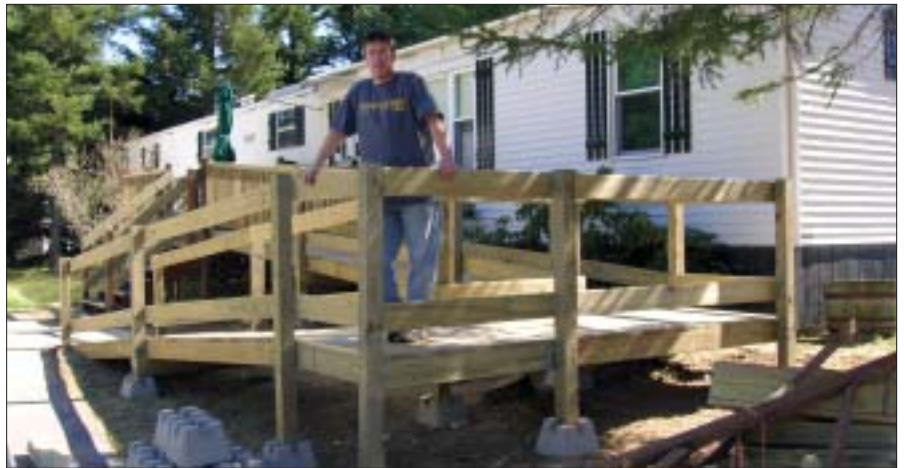
Dan Trembley stands on the completed ramp.
