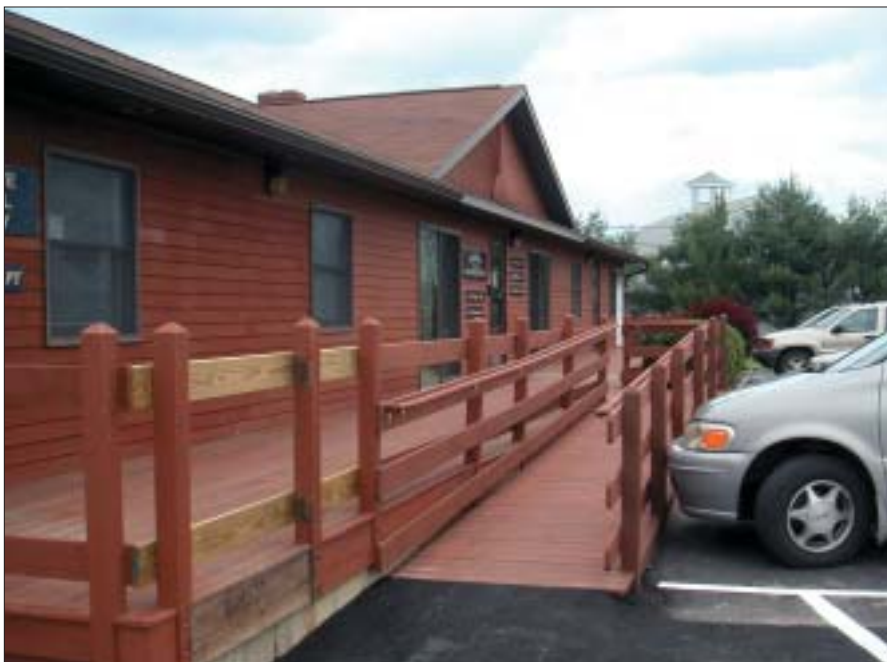
The entrance to Northeast Pain Management has a new handicapped-accessible ramp.
