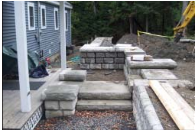
A Redi-Rock retaining wall was installed behind the cottage.
