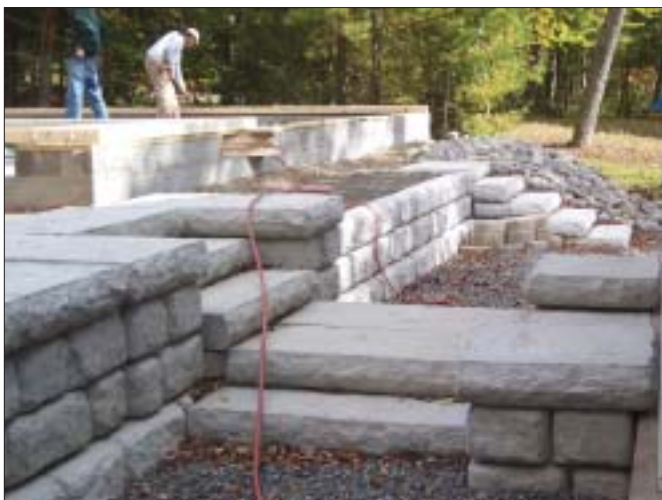
The retaining wall with the garage under construction.
