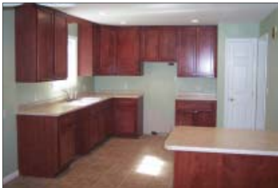
Ms. Dragomir's kitchen with all-new cabinets, before the stove was put back in place.
