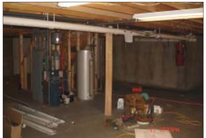
Drew's basement before work began on his dream.
