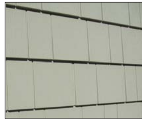
The cedar shake vinyl siding, installed by Ron Michaud, will never have to be painted.
