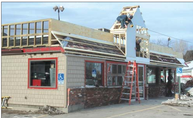
The Governor's Restaurant job in progress.
